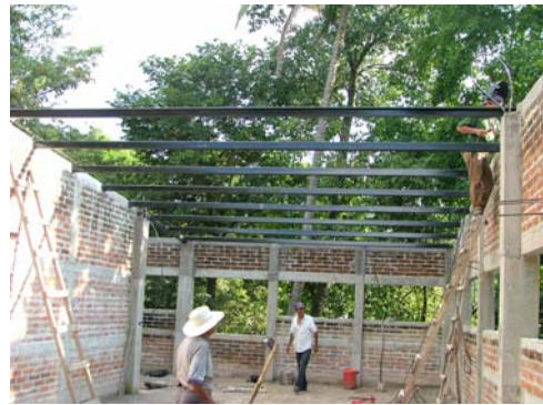
New Church construction
